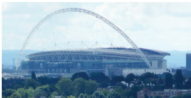
Lasnek HDRF cable tray installed at Wembley Stadium
